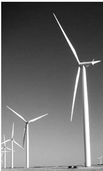
LEFT: Wind turbines located at Horse Hollow Wind Energy Center outside of Sweetwater.
